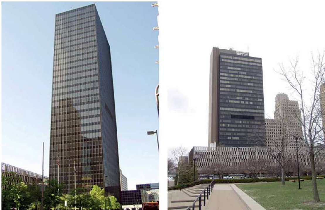
Fuente. NIST TIR 7412 - Evaluating Positive Pressure Ventilation In Large Structures: High-Rise Pressure Experiments. Vistas frontal y trasera del edificio
